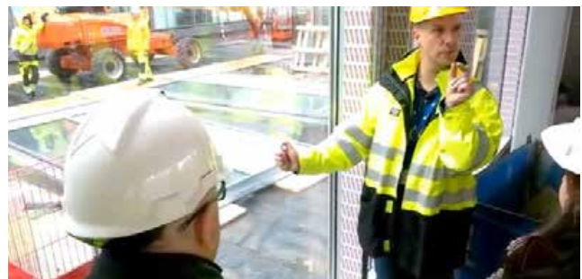
Visit to the Mother-and Child Hospital in Bergen while under construction. This hospital is an outstanding example of modern building materials, new techniques and multicultural labour which demands language competence and cultural understanding
