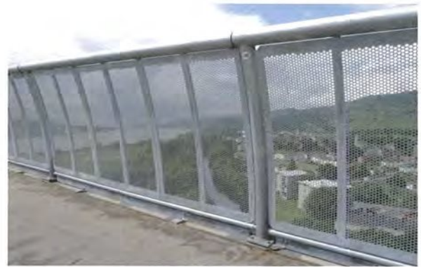
Figure 5b: Parapet over Old Dumbarton Rd
