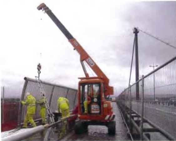
Figures 7a and 7b: Miniature crane operating from cycleway
