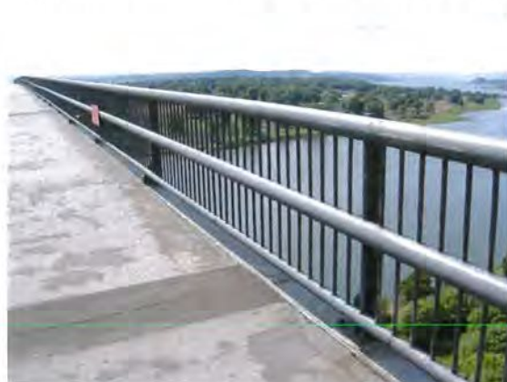
Figure 3a: Original Parapet
