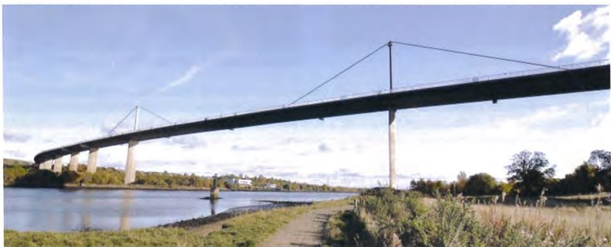
Figure 1: Erskine Bridge with the new parapets installed
