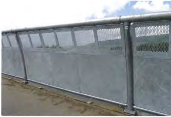
Figure 5a: Parapet over railway
