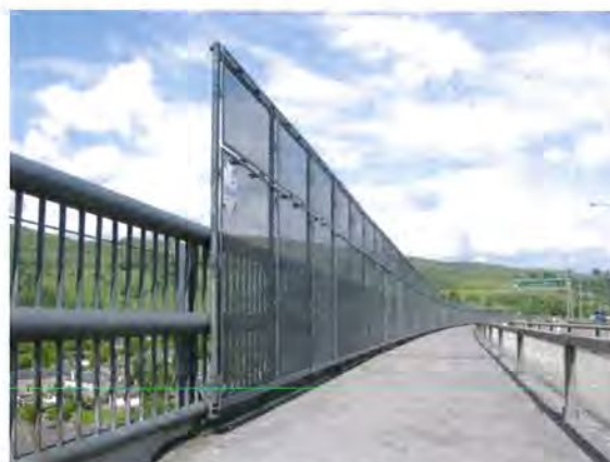
Figure 3b: Mesh screen over Old Dumbarton Rd
