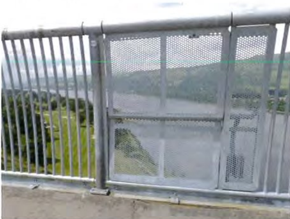
Figures 6a and 6b: Gate for access to maintenance gantry
