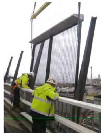
Figure 8: Lifting in of panels
