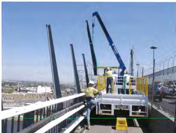
Figure 7: Placing of Posts
