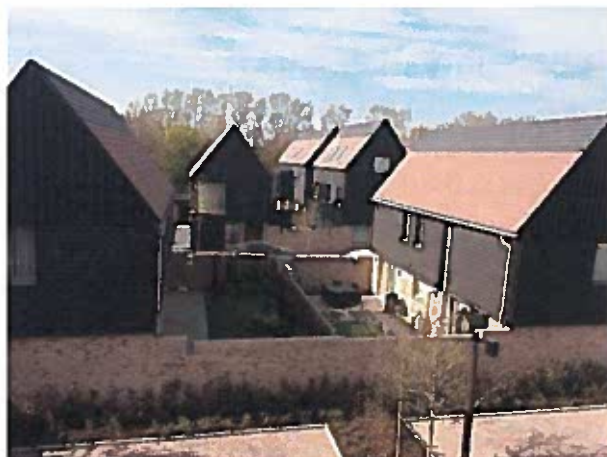
Privat hage, Abode at Great Knighton, Cambridgeshire Proctor & Matthews Architects
