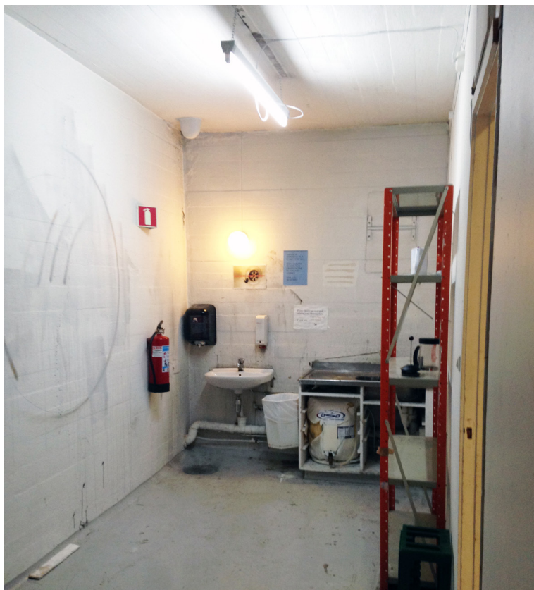
ROOM FOR NEW TOILET AND KITCHEN
