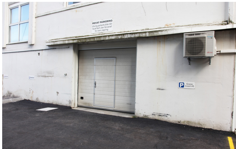
GARAGE GATE FACING PARKING LOT
