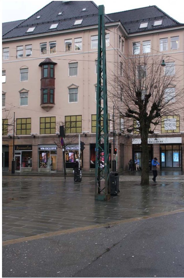
Figure 3 -typical existing OCS pole
