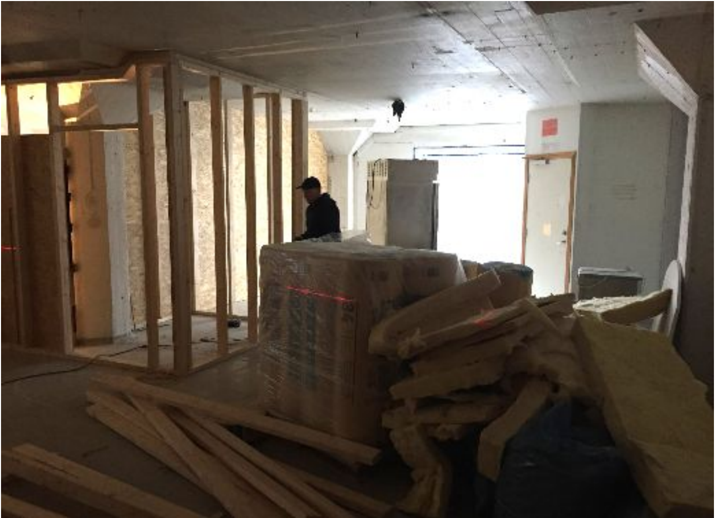
7th Floor - November 9th, Building under Construction
