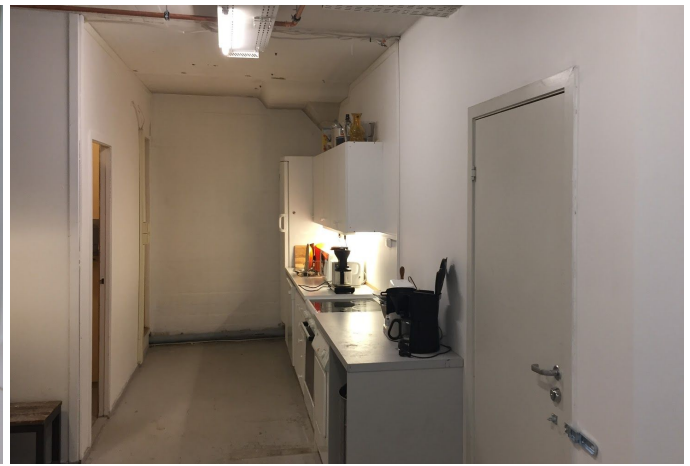
6th Floor - Final Kitchen - October 1st
