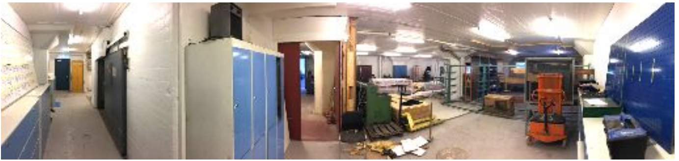
November 9th, Most Equipment in Place
