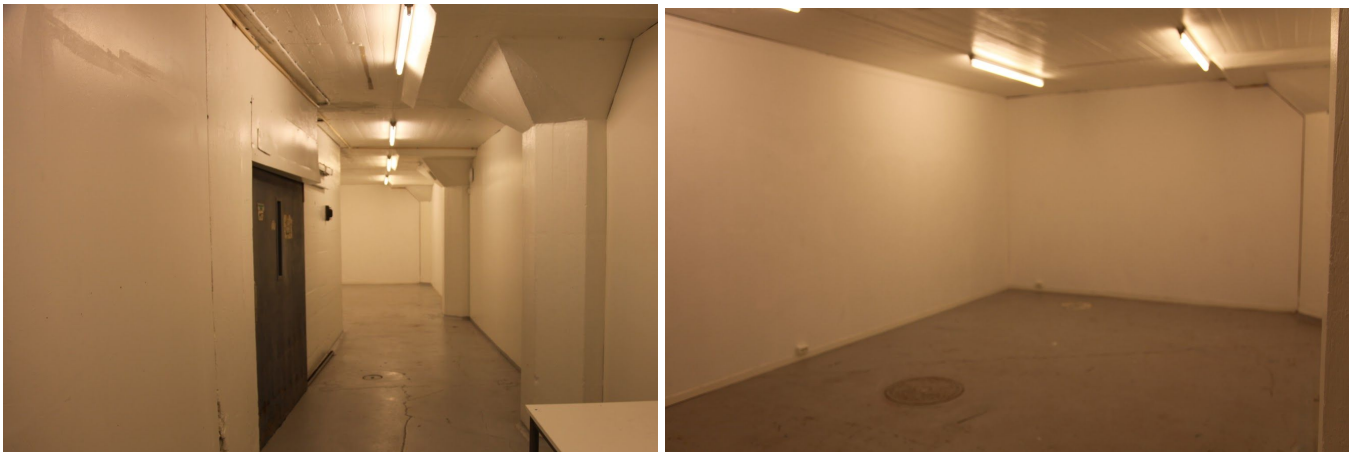
Original walls from inside of front floor.
