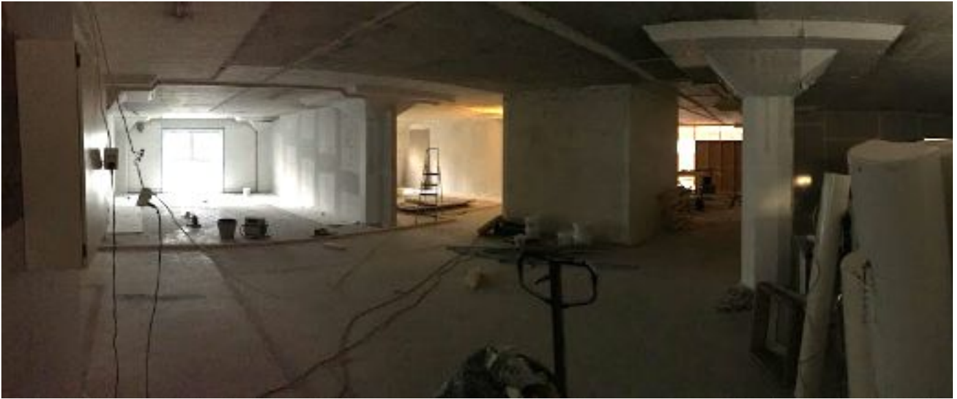
7th Floor - November 9th, Building under Construction
