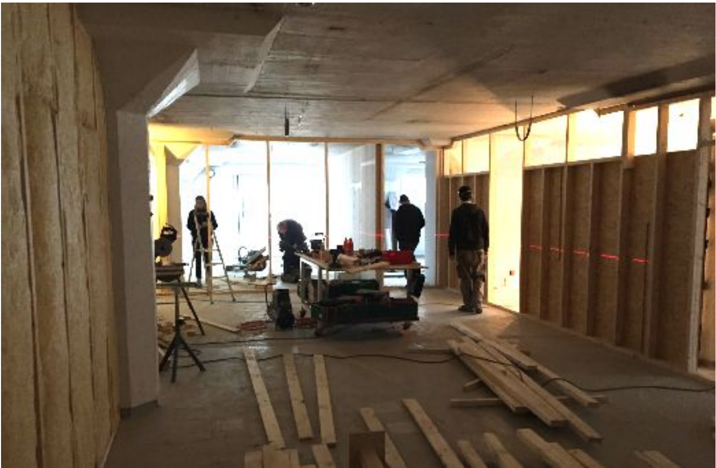
7th Floor - November 9th building under construction
