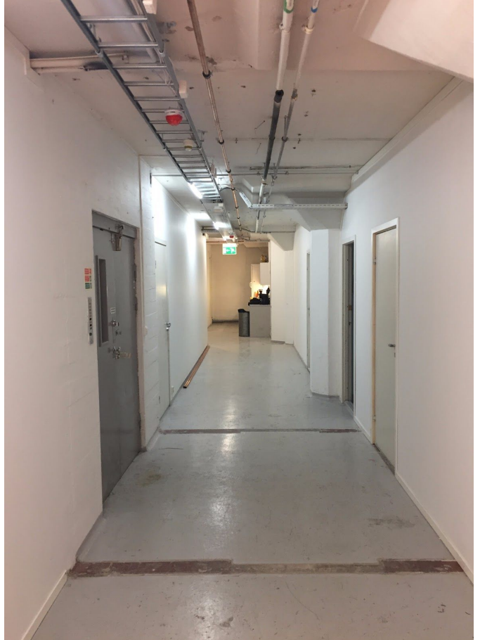
6th Floor - Final construction October 1st
