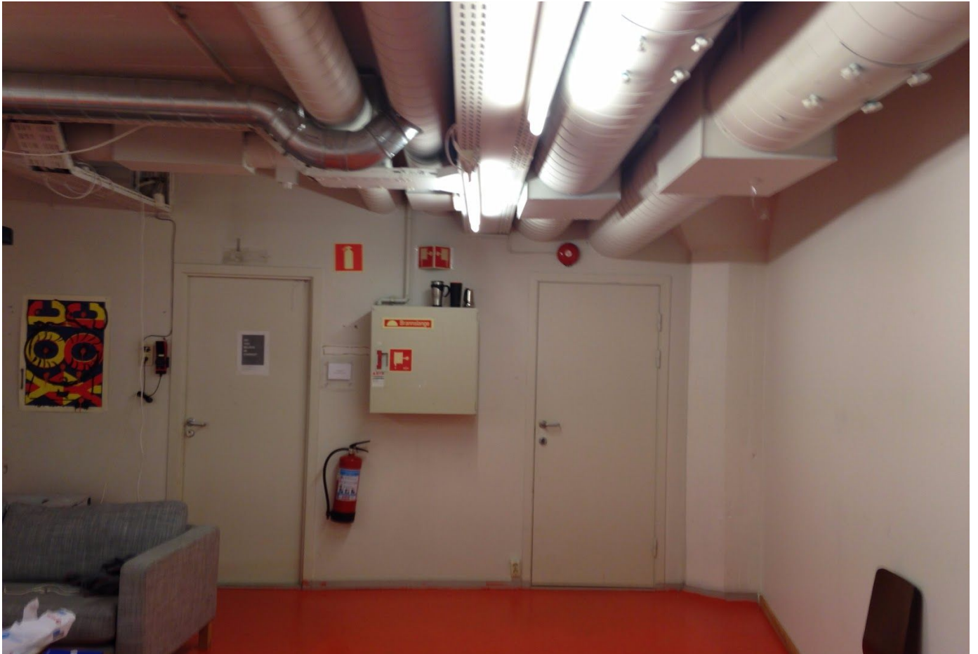
6th Floor - Original studio floor for Khib professors
