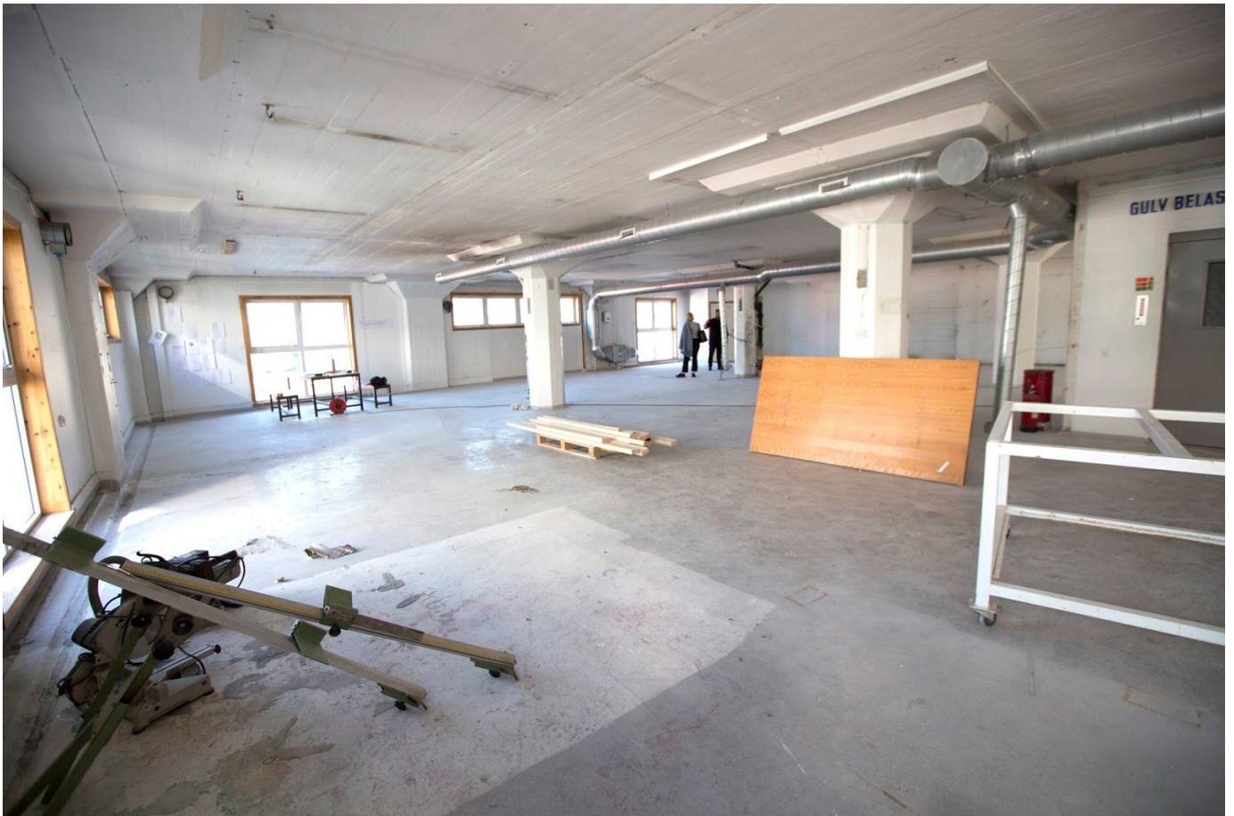
7th Floor after Khib demolishes walls.
